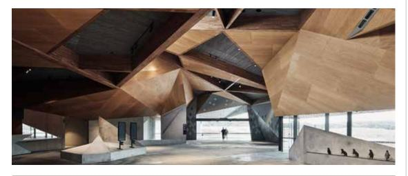
**matilda fireply**<sup>®</sup> is a lightweight, fire-retardant (Group 2 certified) plywood. It is ideal for use as wall and ceiling linings in buildings and projects where improved resistance to fire is required.
