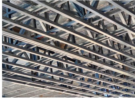
Outdoor ceilings subject to external wind pressure are framed with Studco top hats for maximum strength.
