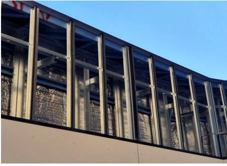
Studco's technical team engineered a structural framing solution using Studco Steel Stud & Track products.
