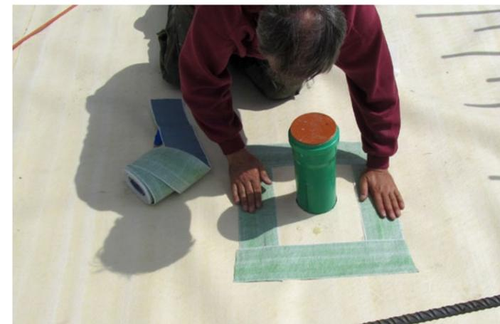
Internal jointing detail with **SikaProof® Tape -150**
