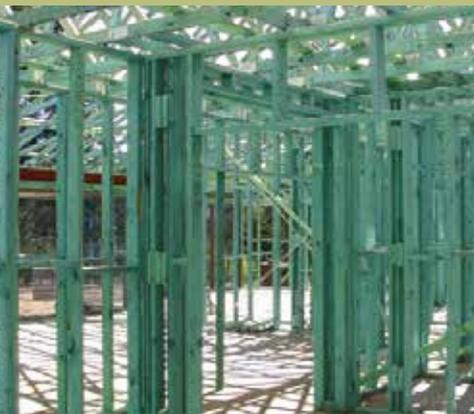
**Treating wood to improve its longevity or reduce maintenance is almost as old as the use of wood itself. Today, pine treated by one of a range of preservative processes is the material of choice for a wide range of internal and external applications.**
