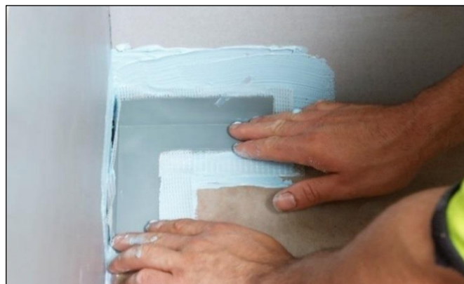
Installing Elastoproof Prefabricated Corners
