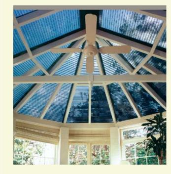
Maxiview® Roof Shutters can be fitted to flat, curved or sloping glass roofs and can also operate uphill.
