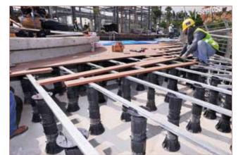
VersiJack® provide stable support for installation of decking
