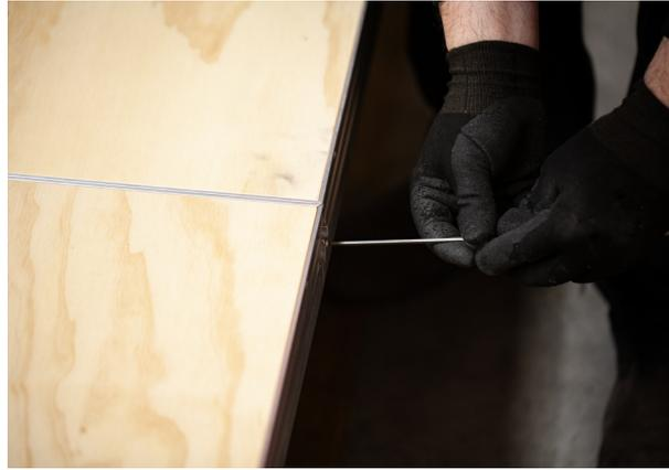
Lock the Klemm-fix Connector with the Allen Key Tool, Hand Tighten.
