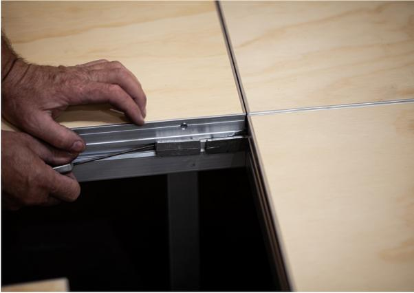
Insert Klemm-fix Connector the correct way up, going in just half way on Interior Podiums or the full way on Exterior Podiums.
