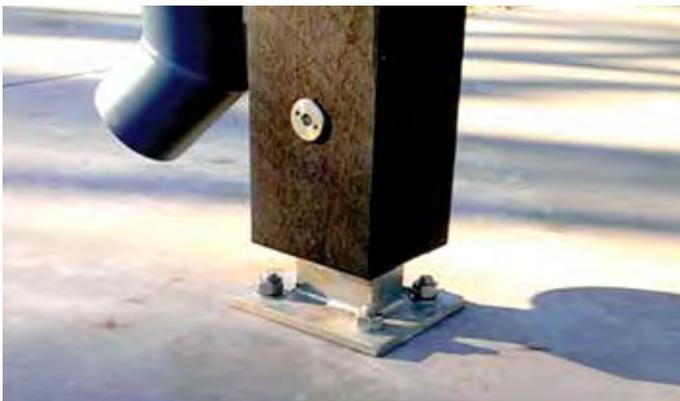
TIMBER BOLT-DOWN TO SLAB
