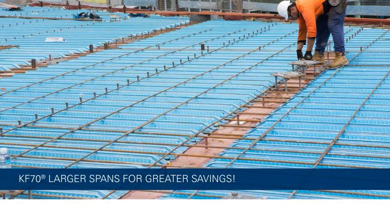
Fielders KF70® is a market leading steel formwork solution for composite concrete slabs in concrete and steel-framed construction. It's the answer to increased market demand for a lightweight profile capable of large spans. The KF70® profile displaces 26mm of concrete from the total slab depth to achieve a lightweight slab.
