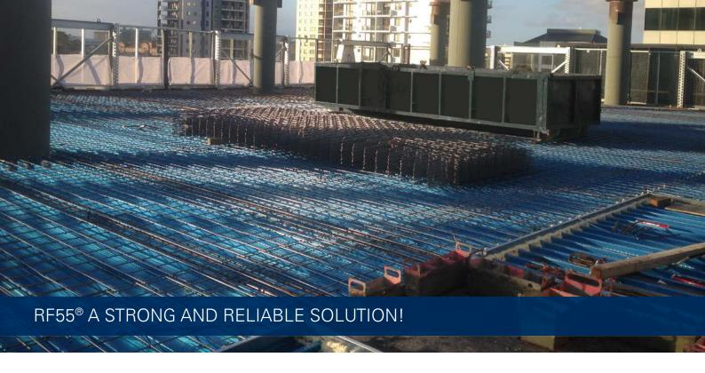
Fielders RF55® is a traditional flat pan or 're-entrant' profile, it provides unmatched performance in suspended concrete slabs. Used in both concrete and steel frame construction it utilises patented technology to achieve superior spanning capabilities, less deflection and greater composite strength than similar re-entrant profiles.
