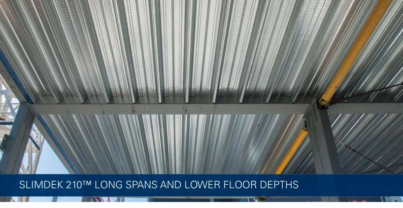
Fielders SlimDek 210™ is a long spanning decking profile capable of achieving unprecedented unpropped spans during construction of up to 7.0m and propped spans of over 10.0m. When combined with Fielders SlimFlor® construction system, floor construction depth can be reduced to as little as 280mm.
