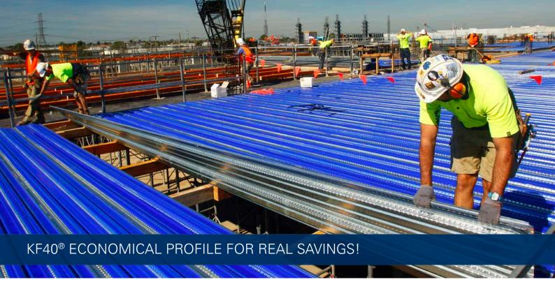
Fielders KF40® is a revolutionary steel formwork solution suitable for concrete slabs in all types of construction. KF40® combines the performance of a traditional flat pan profile with the unmatched economy and concrete saving of a trapezoidal deck.
