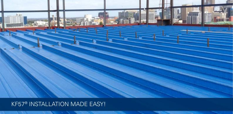
Fielders KF57® provides steel formwork solutions suitable for composite concrete slabs in concrete and ramed construction. Light, easy to use, steel decking designed to combine with a concrete slab to produce a composite concrete slab system. KF57® incorporates an improved deck profile with deeper pan stiffeners.
