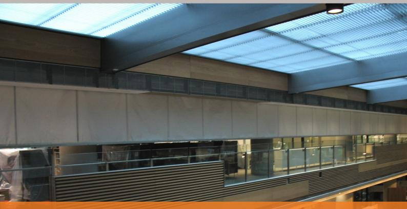
Built for distance, the Supercoil long span vertical smoke curtain is tough and reliable, resisting pressures up to 100Pa (50m2 system) and 50Pa (100m2 system) when fully deployed
