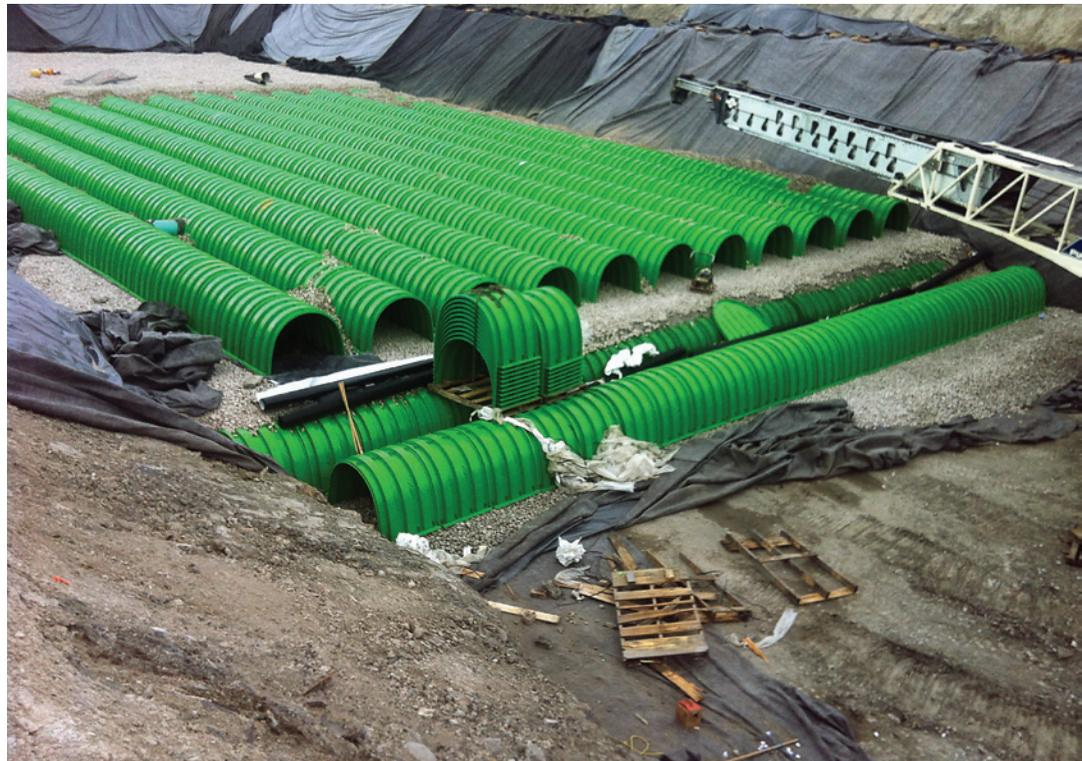
Triton SWS' unique double-stack design allowed developers to create 22,000 cubic meters of storage in a 20m x 70m area for a new retail center in Toronto, Canada.
