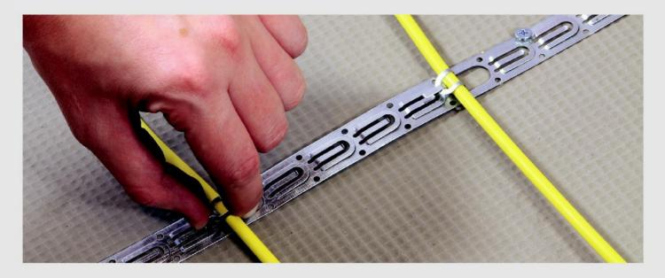
Thermoscreed<sup>™</sup> is a heavy duty 5.5mm underfloor heating system designed for use in concrete screeds and suspended timber floors.
