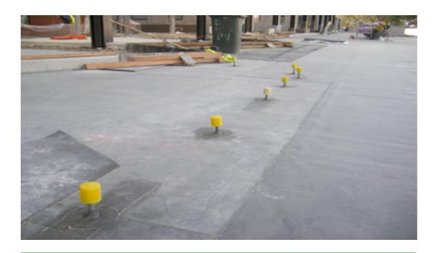
Anchor points for concrete curbing and islands have been detailed & waterproofed using standard Wolfin installation procedures. Over 3,500 square metres of Wolfin were used in this area.
