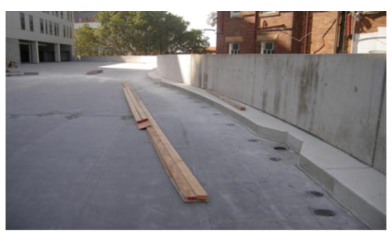
Concrete curbing placed on 5mm Projex Shockmat membrane protection layer
