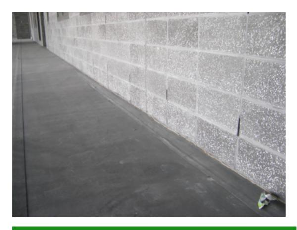
The Wolfin membrane system continues under the block façade to form the cavity flashing
