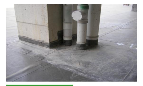
Wolfin IB is welded directly to PVC pipes
