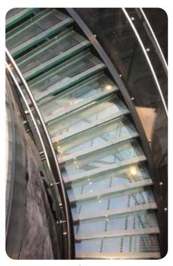
**Stair treads:**39.04mm clear toughened structural laminated flat glass with SGP interlayer
