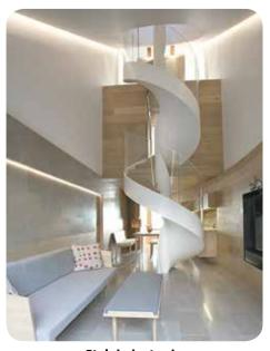
**Stair balustrade:** 15.04mm low iron toughened structural laminated curved glass
