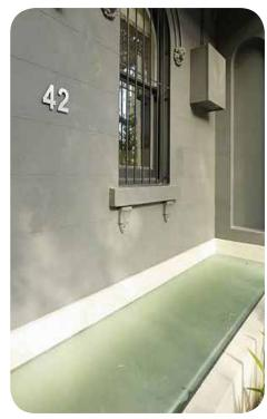
Front entry porch: 37.52mm flat toughened glass with clear PVB interlayers. Antislip frost seraphic frit to top surface.
