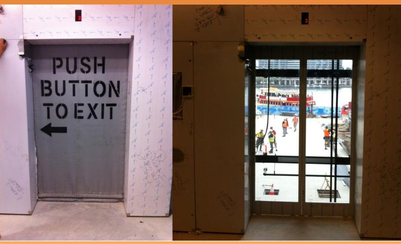
Fiberseal-fs vertical fire and smoke containment screen system can be cleverly used in conjunction with mechanical smoke exhaust systems to reduce opening dimensions, and therefore fan sizes to create a cost effective overall solution
