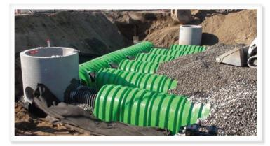
Again, the crew quickly places the chambers – including the innovative Main Header Row that allows for a host of pretreatment options.
