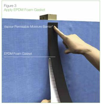
At every vertical joint, fix a continuous strip of EPDM Foam Gasket to the vapour permeable moisture barrier along the stud. This assists to prevent moisture ingress at the sheet joins.
