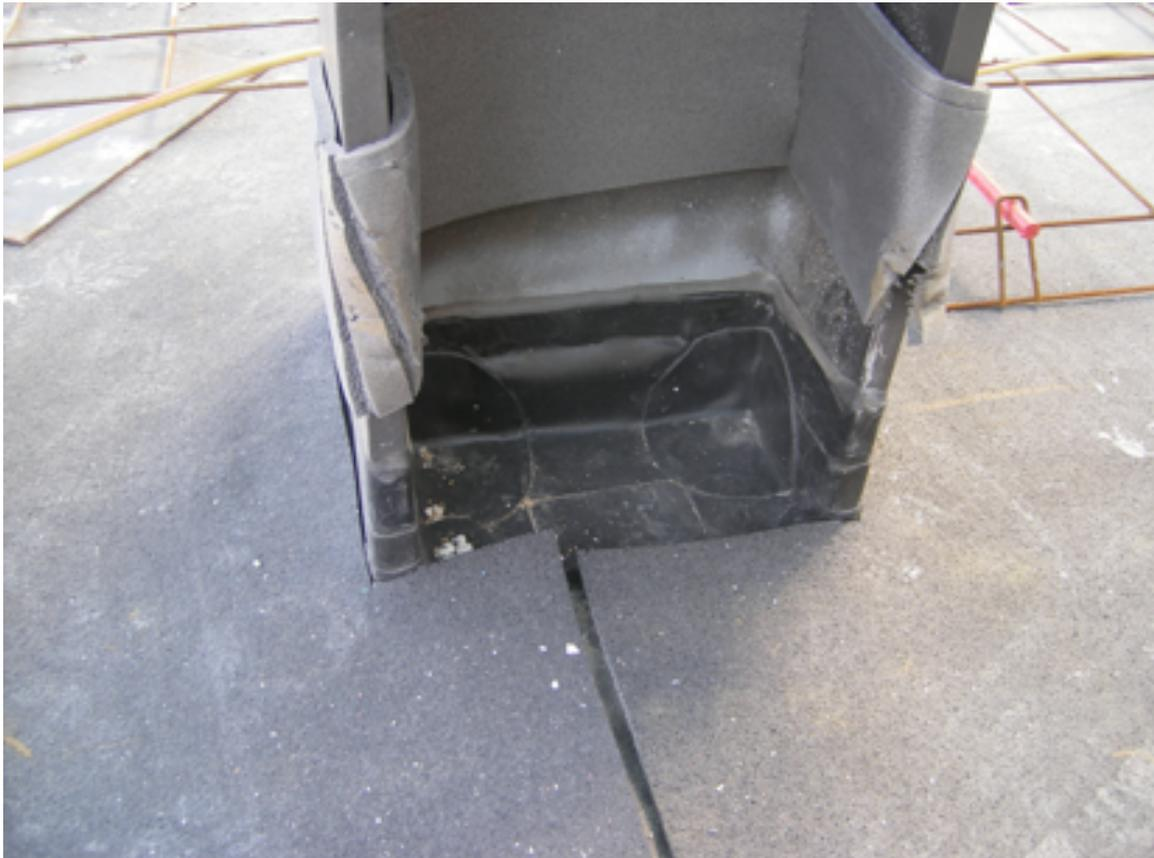
*The Wolfin membrane system is sealed to the steel “H” columns that support the covered walkways.*
