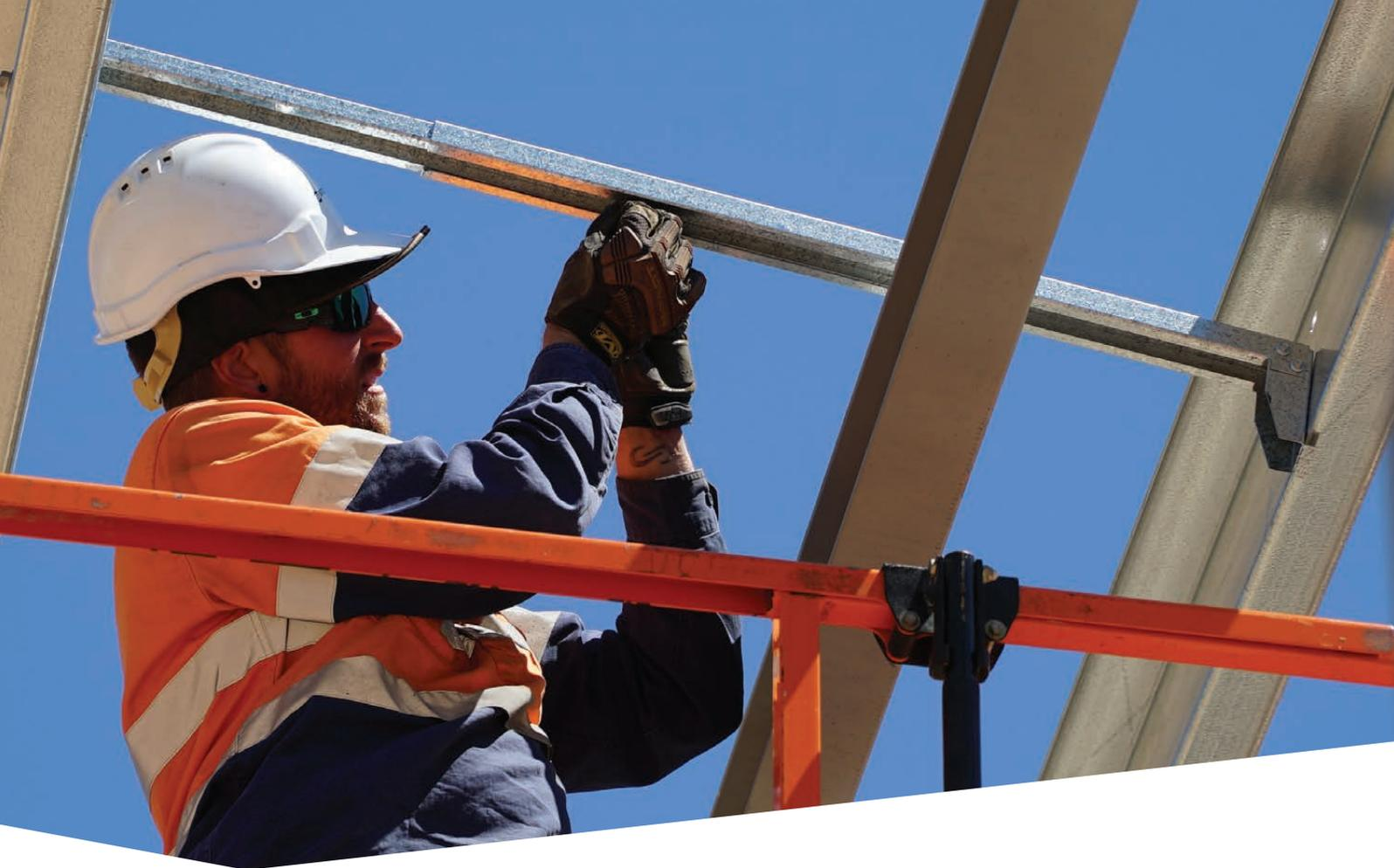
**SUPABRIDGE™ bridging sections are spaced at a maximum 1500mm centres along the SUPAPURLIN® length.**
